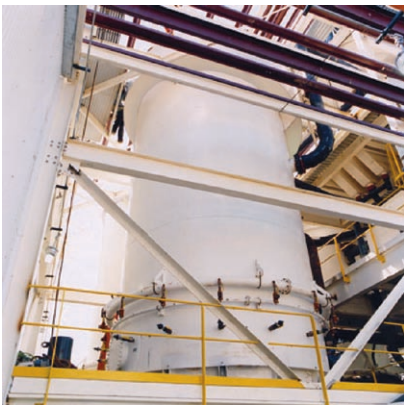
Figure 7. Eriez CoalPro column flotation cells illustrating froth washing system.
